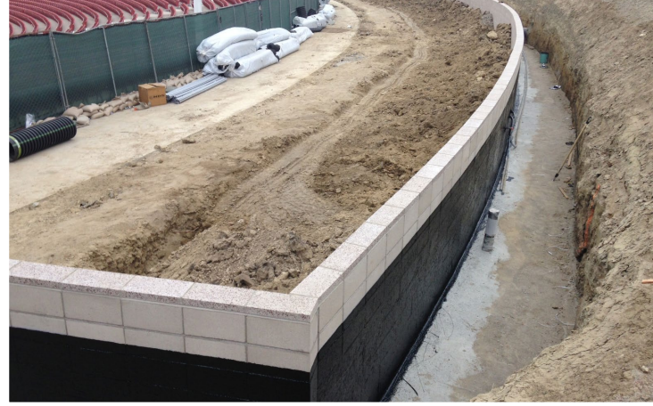
PROJECT: Pacific Amphitheatre, Costa Mesa, CA PRODUCTS USED: TREMproof® 250GC
